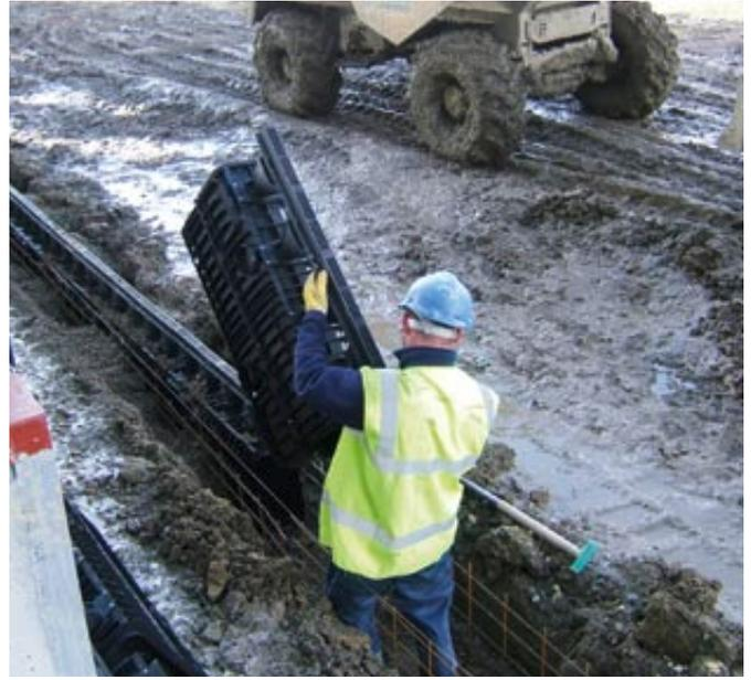
Lightweight elements, installed by one single worker.
